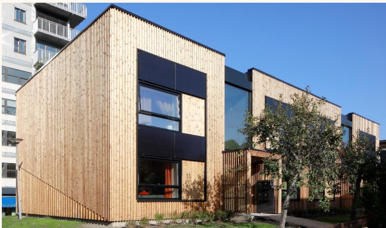
Figure 2. Rehab project at Haugerudsenteret. The PV panels are installed in pairs above the large windows (south façade) and integrated into the prefabricated elements. Image courtesy: Oslobygg.
