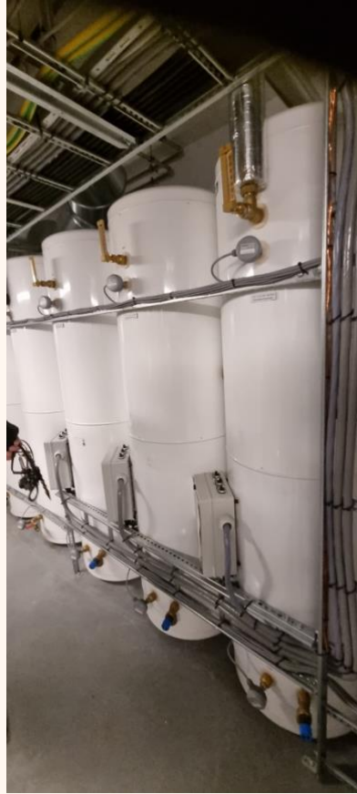
Figure 16. Installed water tanks for short-term thermal storing.
