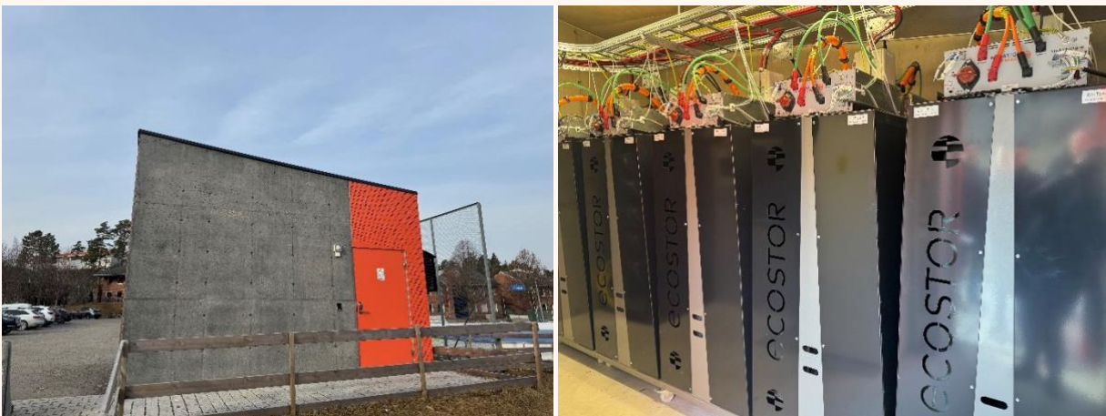
Figure 8. The battery building at Holmlia school seen from the outside (left), and the installed battery modules (right). Photos by Aileen Yang/SINTEF.
