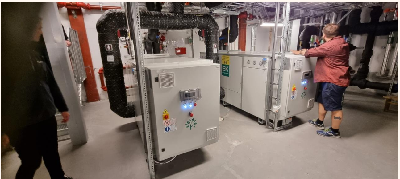
Figure 15. Installed CO 2 heat pump at the Voldsløkka school.
