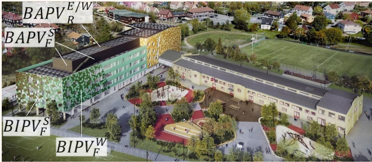
Figure 11. Overview of the ARV demo Voldsløkka school with PV systems on the roof and facades of S-building (on the left): Image courtesy of Veidekke [16].
