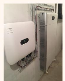
Figure 13. 15 kWh battery unit and battery inverter for 1 of the 19 housing blocks
