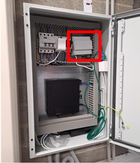
*Figure 50. Prototype of advanced control and monitoring system for HVAC assets. Photo: IREC*
