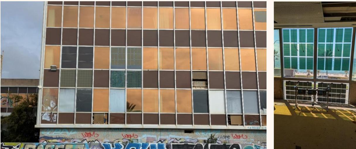
**Figure 24.** Images of the BIPV testing in GESA building in Palma. External view (left) and internal view (right)
