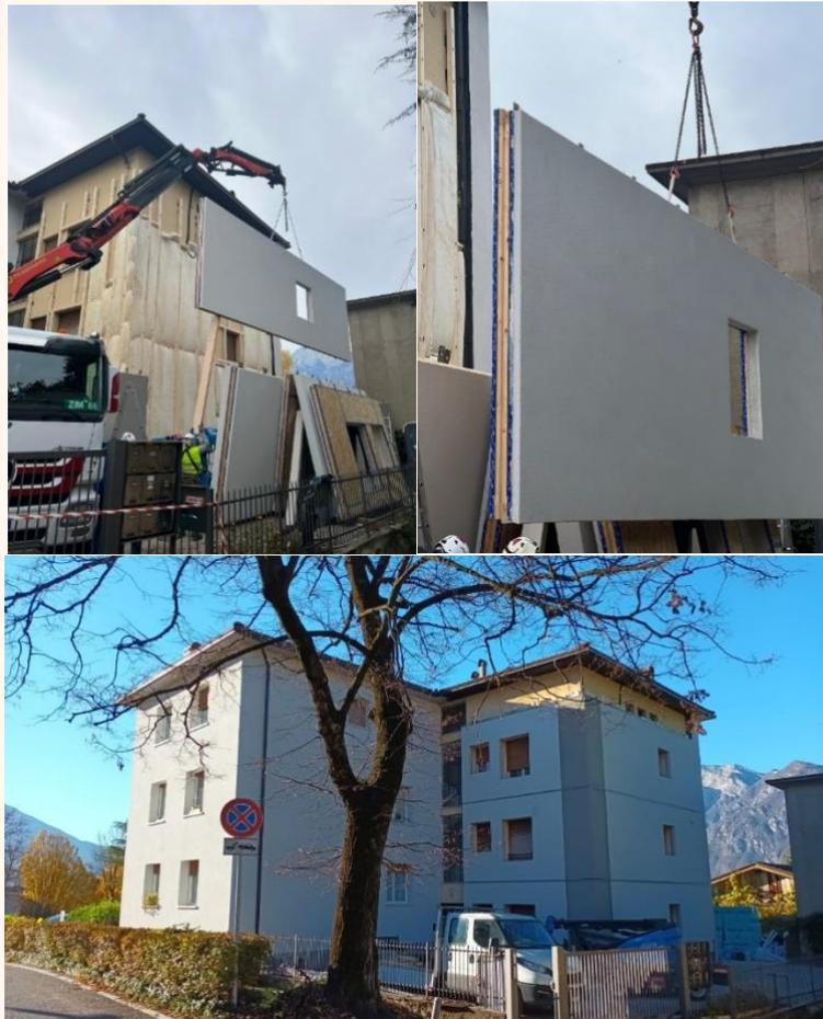
*Figure 21. Installation Phases of Renew Wall prefab-kit, Trento - Povo Demo*
