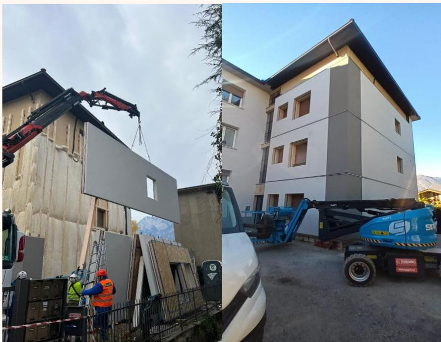
*Figure 29. Before and after the installation of the “Renew Wall” retrofit kit in Povo.*
