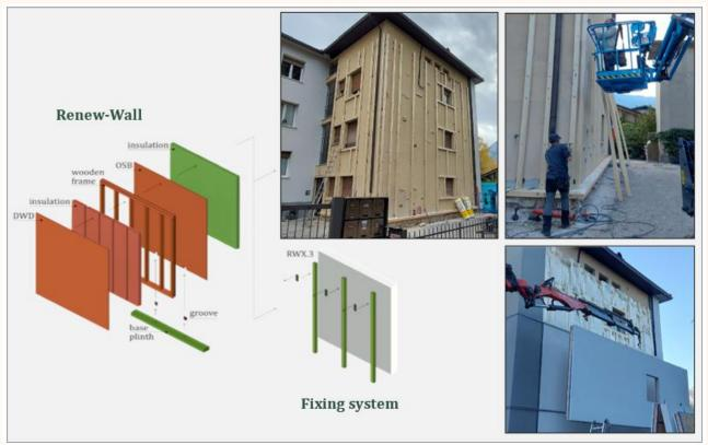
*Figure 22. System for fixing the Renew-Wall to the Existing Building facade: schematics of the system (on the left and bottom center); photos of the installation - Demo Project Trento, Povo District (on the top centre and right)*
