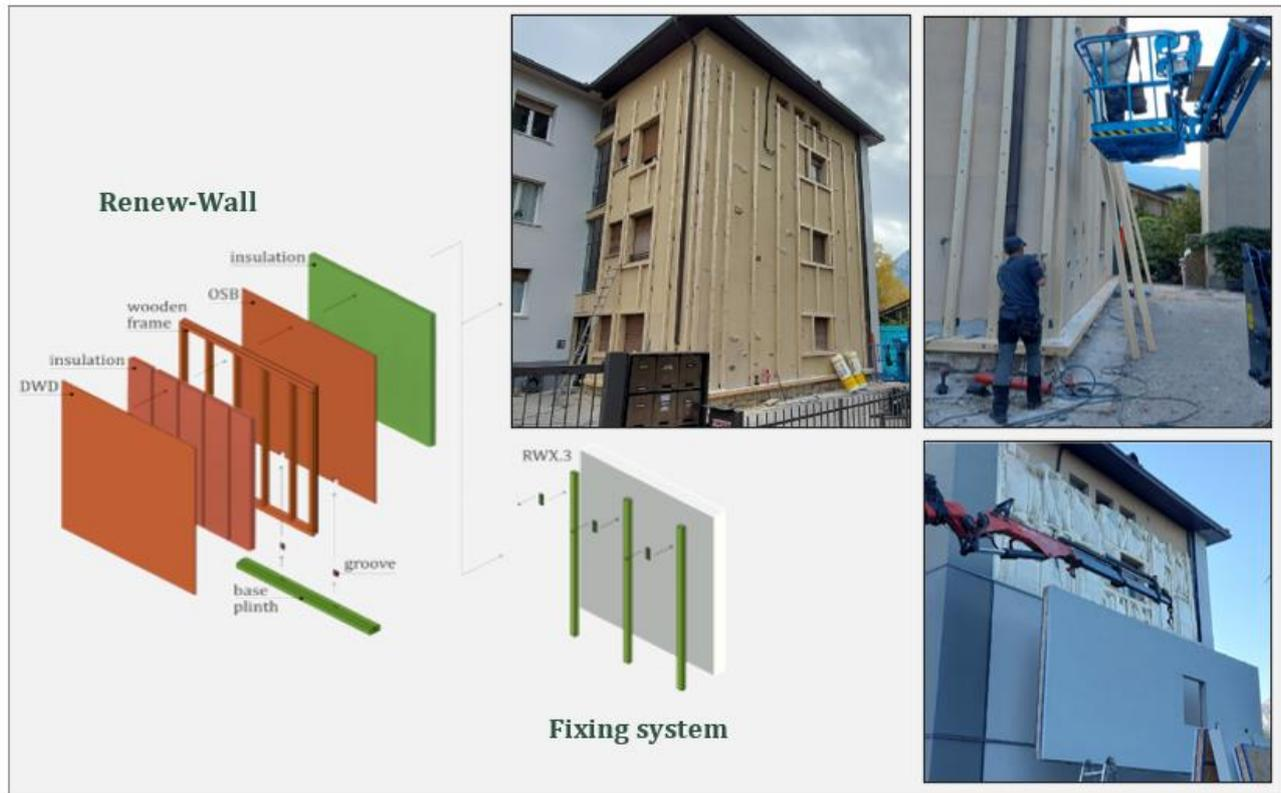
**Figure 22.** System for fixing the Renew-Wall to the Existing Building facade: schematics of the system (on the left and bottom center); photos of the installation - Demo Project Trento, Povo District (on the top centre and right)
