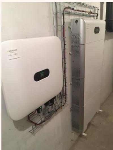
*Figure13. 15 kWh battery unit and battery inverter for 1 of the 19 housing blocks*
