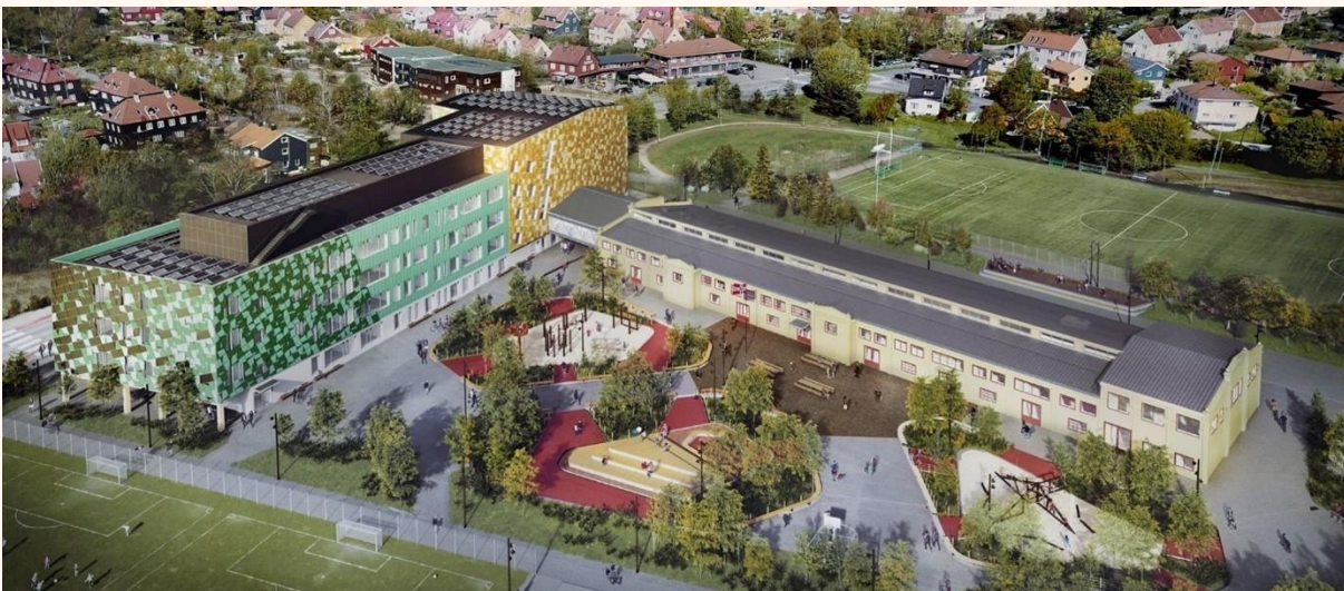
Figure 7. Aerial view of the Voldsløkka school project
