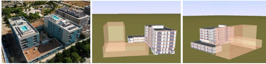
Fig. 1. The Metrovacesa highly efficient multi-family residential building (left) (source: Metrovacesa). Block 1 with NE orientation (middle) and block 2 with SW orientation (right).
