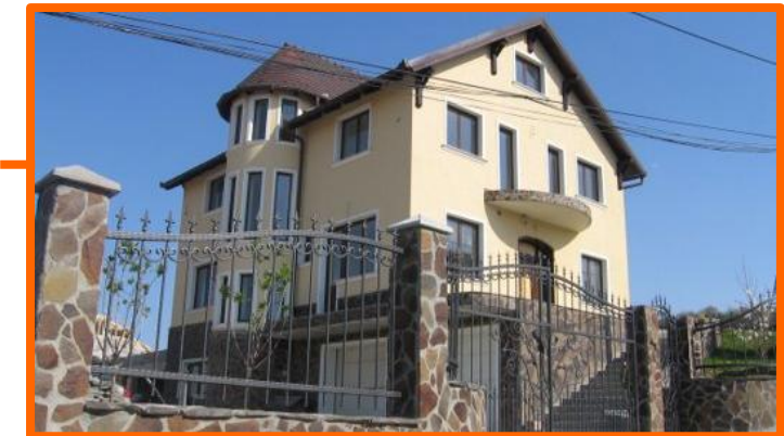
Single family building - Oredea (Romania)
