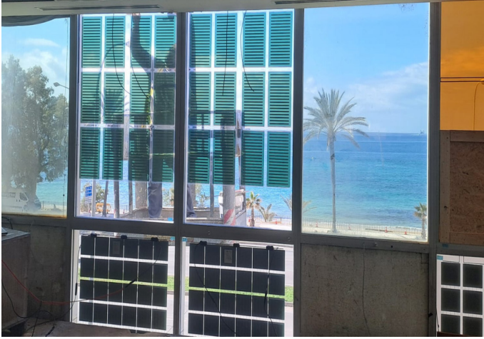
Installation and testing of PV in Palma Source: Metrovacesa
