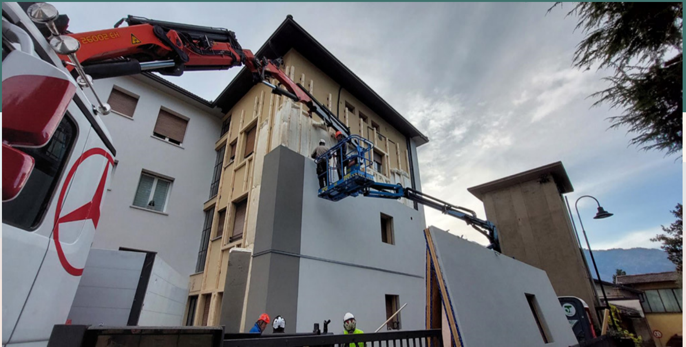
Installation phases of the Renew Wall panels on the residential Existing Building in Povo District. Source: UNITN.
