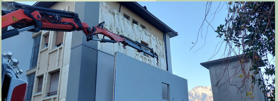
Installation phases of the Renew Wall panels on the residential Existing Building in Povo District. Source: UNITN.
