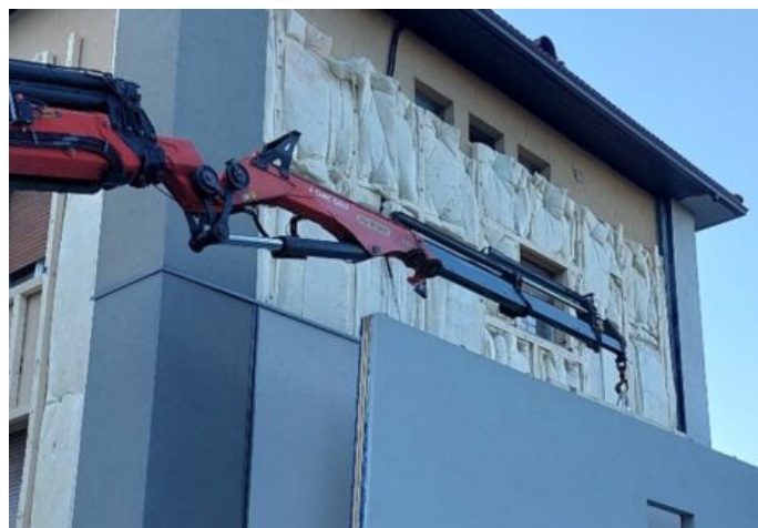
Renewal Wall panel installation Source: UNITN.
