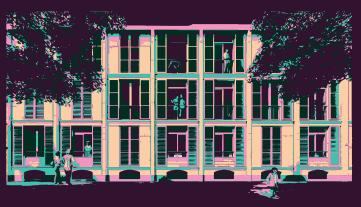
This innovation aims to make buildings adaptable to external climate conditions through bioclimatic elements to regulate ventilation in summer and heat conservation in winter. CO2, temperature, and humidity sensors installed in each room will control motorized windows to maintain optimal comfort levels. It reduces energy losses during air renewal and lowers energy demand, automating the system to minimize user effort.
