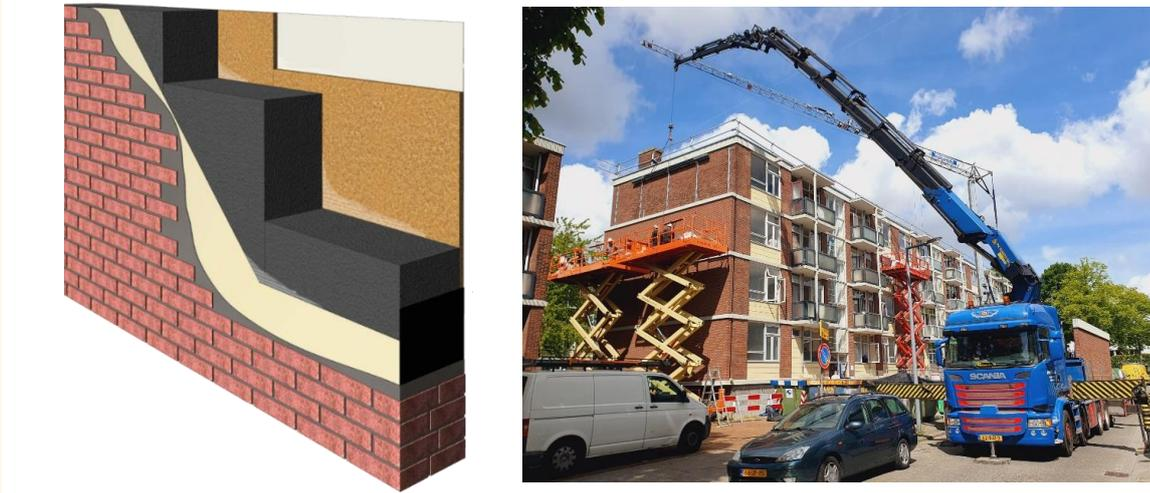
*Figure 2. Left: Prefabricated facade panel design by Rc Panels showcasing its five layers: polyester, OSB, EPS in various thicknesses, polyester, and a finishing stone slip layer. Right: retrofitting of Hoge Kampen flats with a prefabricated building envelope. Source: Rc Panels*
