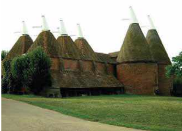
Figure 18: Wind cowls able to move with the wind changing direction in a beer brewing of Kent (England) [25]
