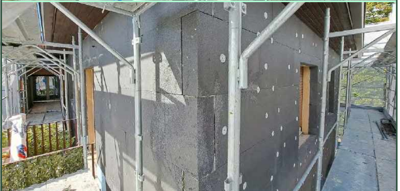
Installation of EPS insulation (ETICS)
