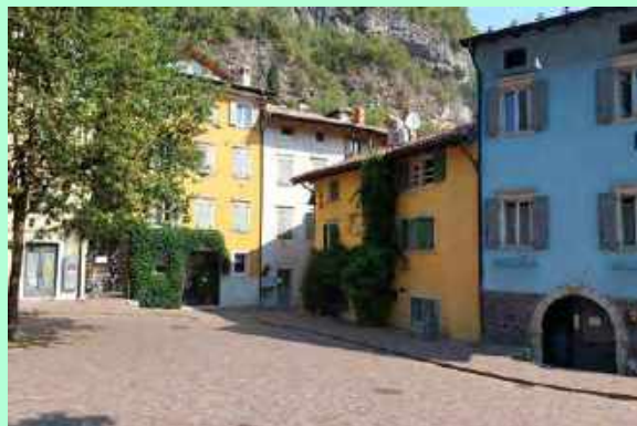
2. View of historic buildings
