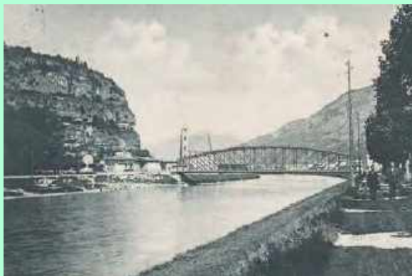
5. San Lorenzo iron bridge, 1924
