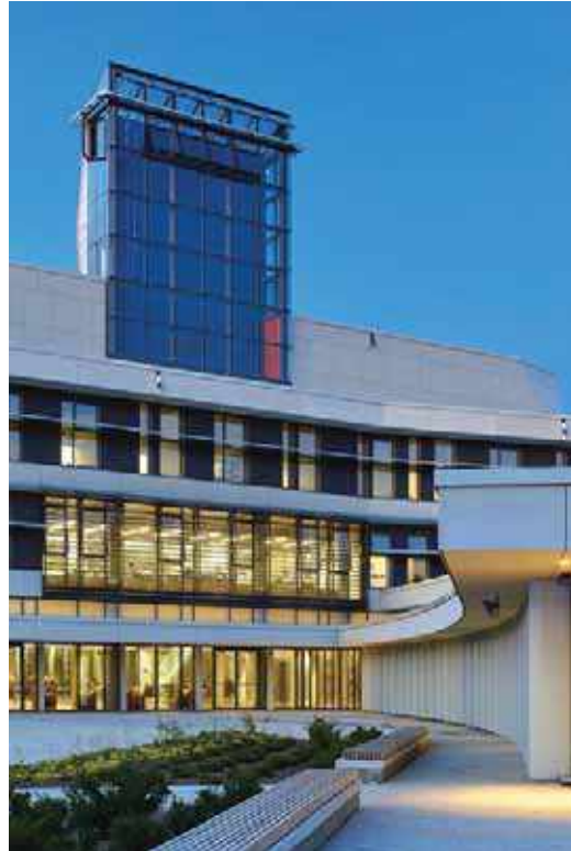
Figure 31: McEwen Graduate Study & Research Building in York University (Toronto, Ontario, Canada) – a solar chimney for facilitating NV [35]
