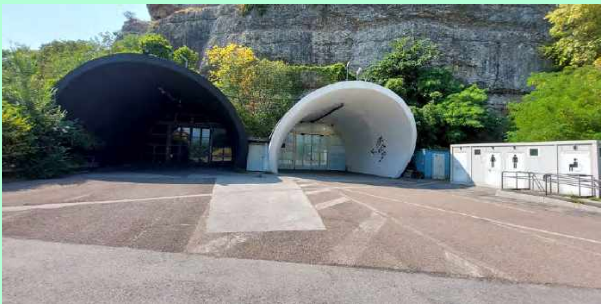
4. Exterior view of the two disused road tunnels - north side
