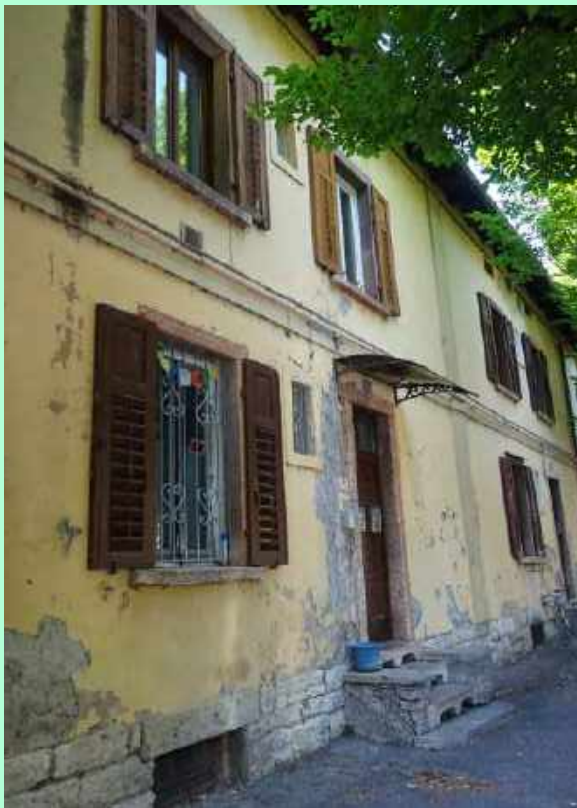
3. Access with steps to building in Verrucca street
