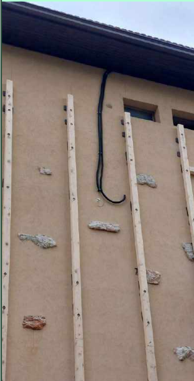
Installation of sensors in RW panel for envelope monitoring
