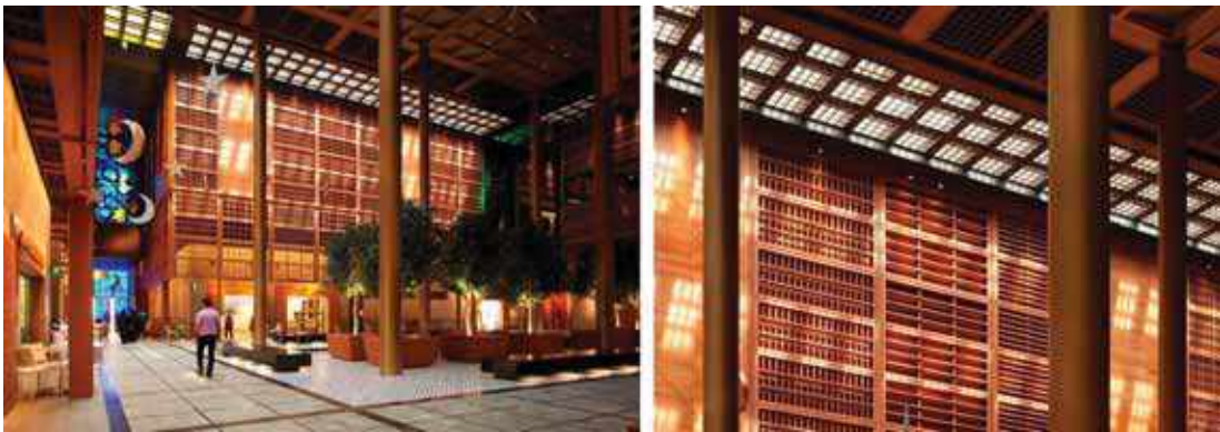
Figure 3: “Abu Dhabi Central Market” (United Arab Emirates, UAE). Resembling the traditional Islamic art of coffered roofs, the covering is able to adapt to different sunlight conditions, with natural cooling when allowed by outside conditions [7], [14]
