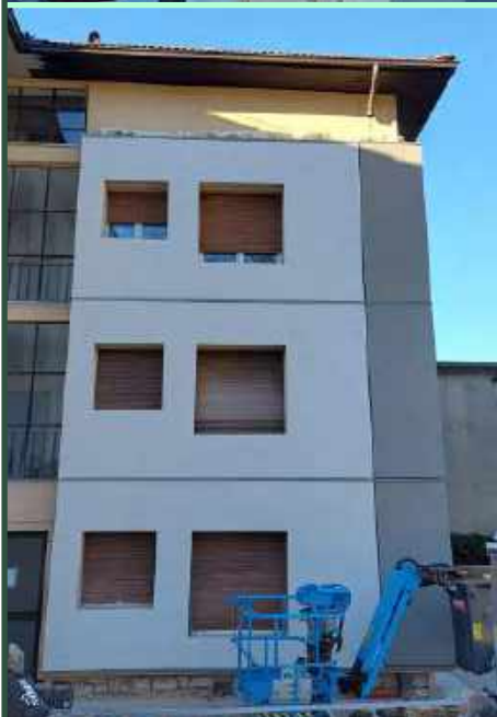
Installation of RW panels
