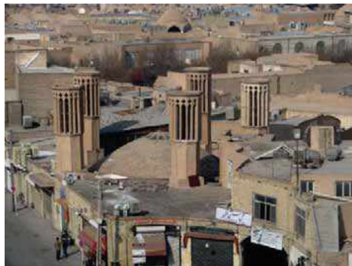
Figure 14: Yazd (Iran) – traditional wind towers [25]
