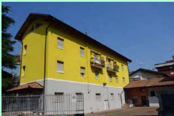
4. Building in Doss Trento street
