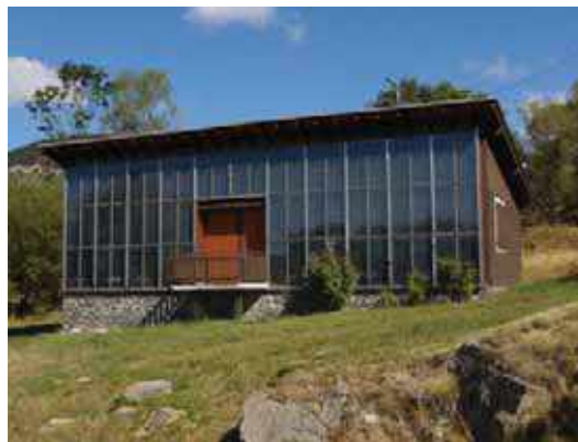
Figure 29: Trombe wall in Vivienda Trombe (Odeillo, France) [34]
