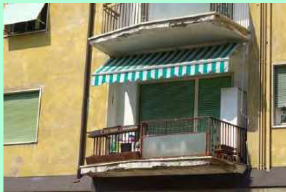
3. Detail of a building of social housing
