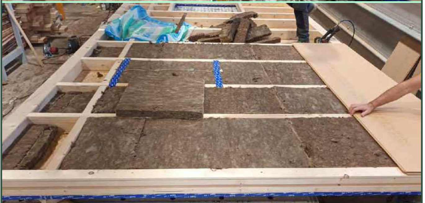
Installation of sensors in RW panel for envelope performance
