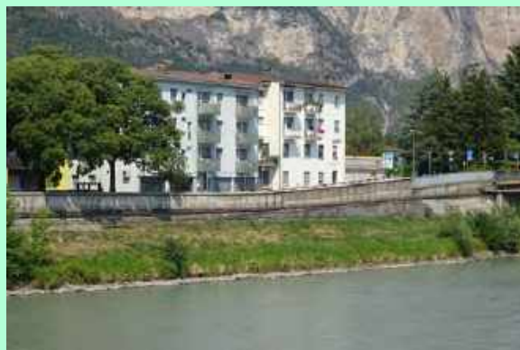
5. Recently renovated buildings of social housing
