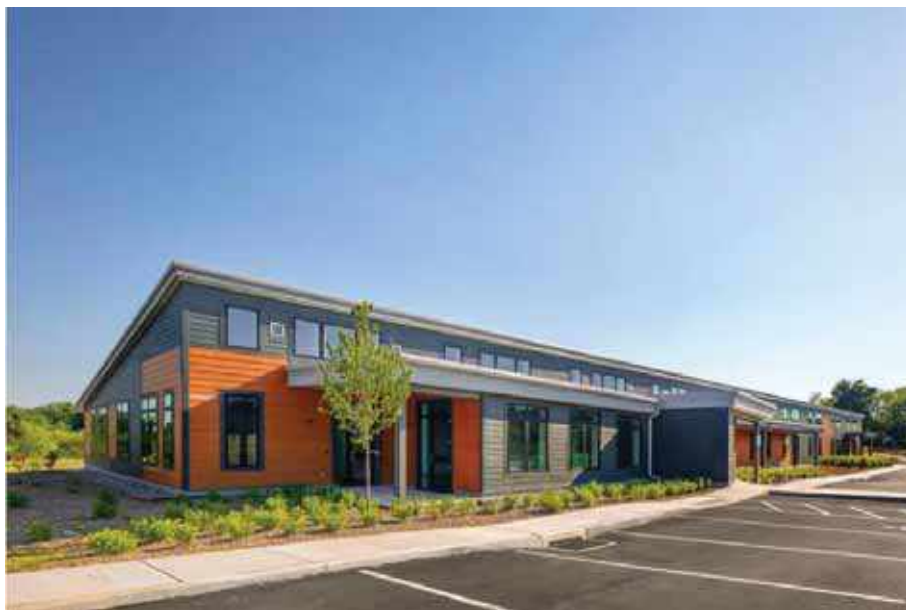
Figure 4: “Sustainable Energy Fund Office Building” in Schnecksville (Pennsylvania, USA). The building orientation and windows’ design allows to take advantage from shade, sun and daylight, minimizing the loss of energy. It also uses a roof photovoltaic array. It is planned to generate 130 % of the required energy [15]
