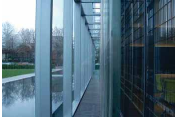
Figure 40: Double-skin façade of the university building considered by Azarbayjani study [106]
