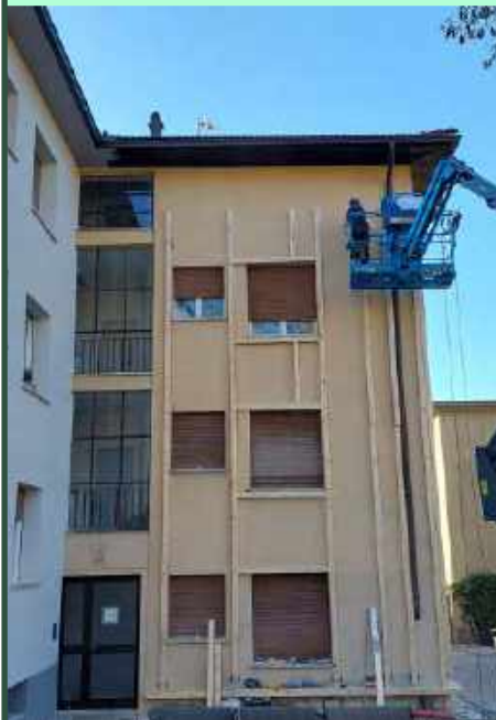
Installation of RW panels
