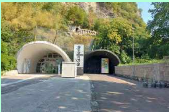
4. Area 3: two disused road tunnels
