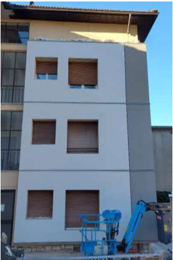
Figure 56. Installation of the Renew Wall panels. Source: UNITN.
