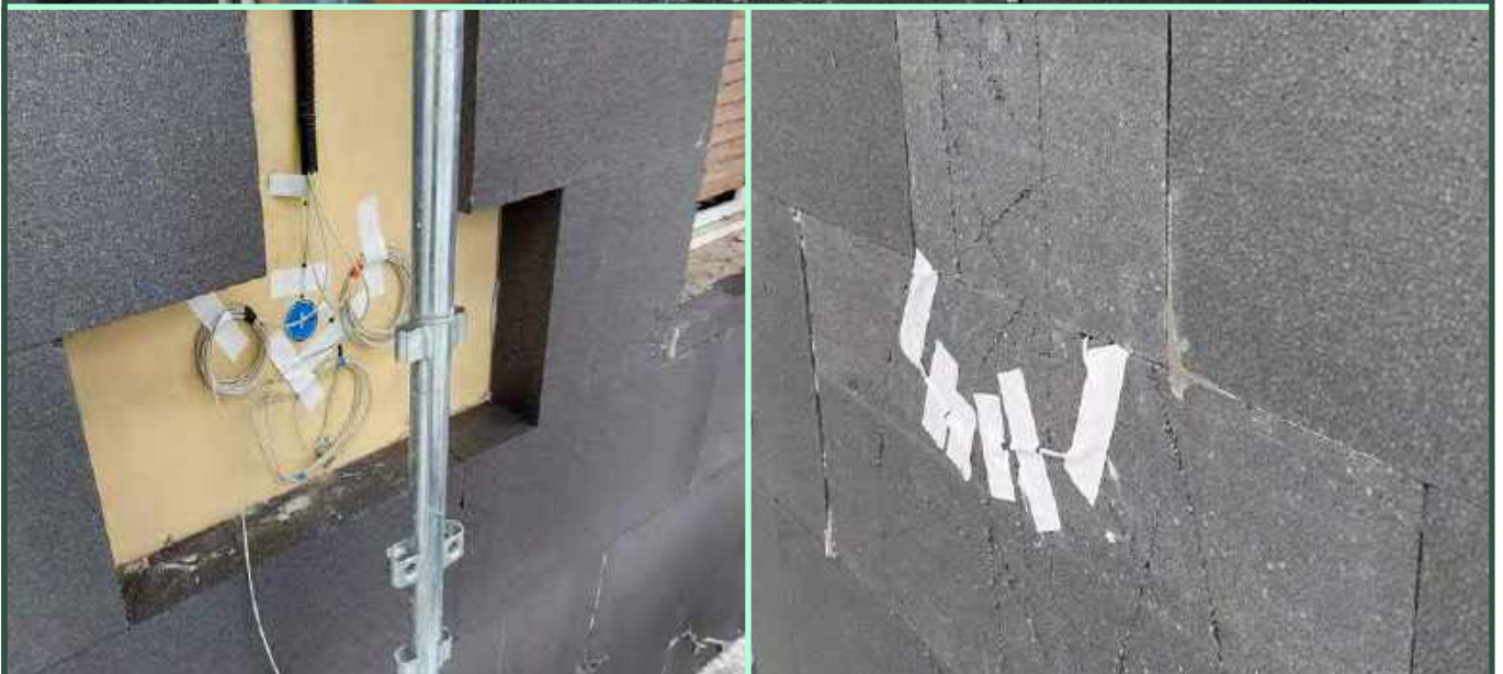
Installation of sensors in ETICS for envelope monitoring
