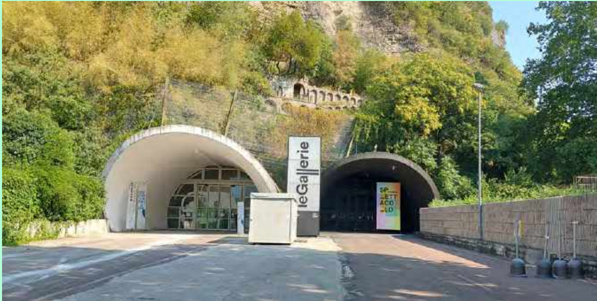
1. Exterior view of the two disused road tunnels - south side
