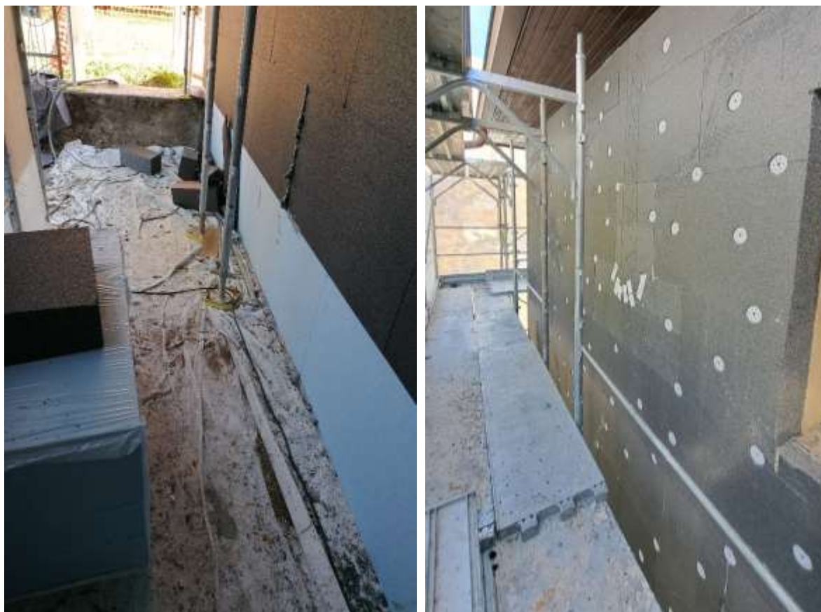
Figure 55. Installation of the EPS insulation. Source: LEVA Srl.
