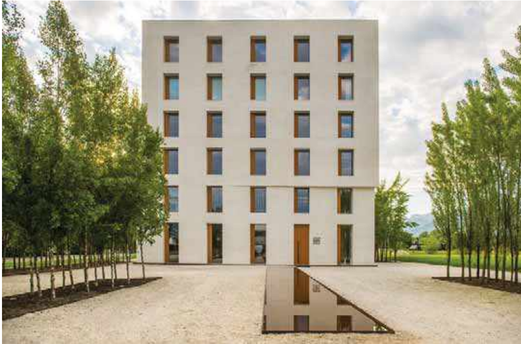
Figure 5: “2226” in Lustenau (Austria). The office building does not use energy sources different than internal gains or solar gains, being able to always maintain a temperature comprised between 22 °C and 26 °C by means of construction techniques, night cooling by means of natural ventilation, proper use of thermal mass and sensors’ support [10], [11], [16]
