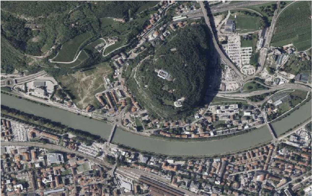
Figure 2. Aerial view of the Destra Adige - Piedicastello district (Source: Google Earth).
