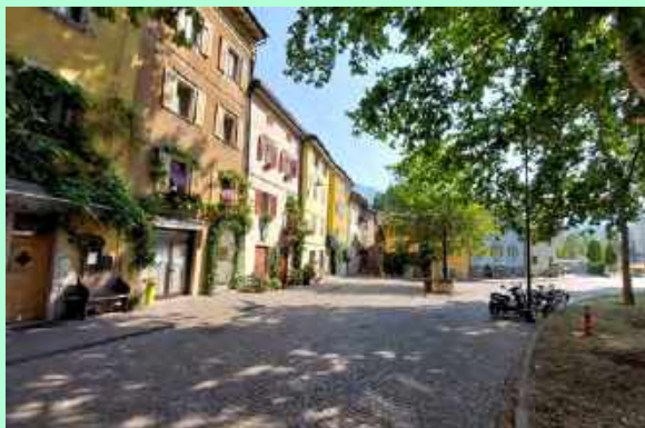
1. View of historic buildings
