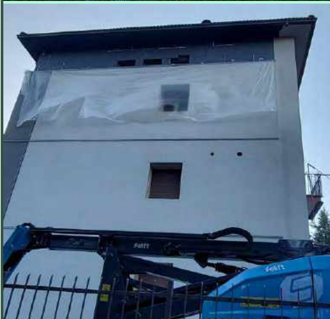
Finishing work at the base and top of the RW panels
