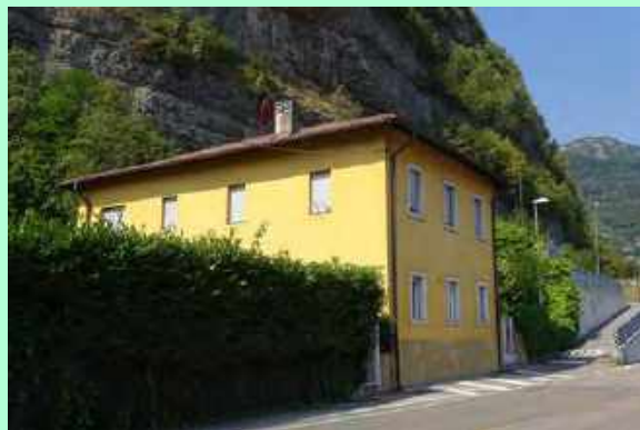
2. Building in Doss Trento street
