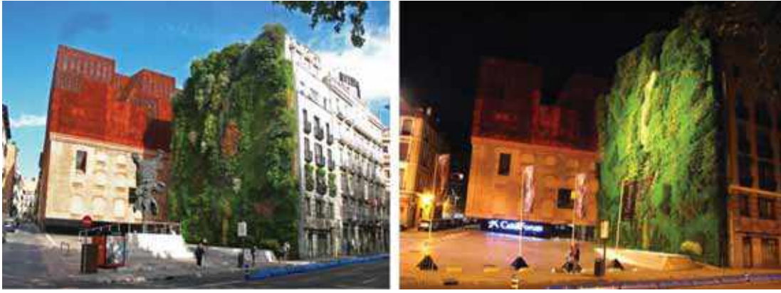
Figure 2: “Caixaforum Vertical Garden” in Madrid (Spain). 250 species of plants grow on a 460 square meters vertical garden, contributing in creating indoor and outdoor thermal comfort conditions [7], [13]
