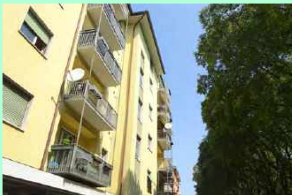
4. Detail of a building of social housing
