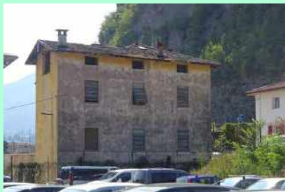
7. Building in Doss Trento street
