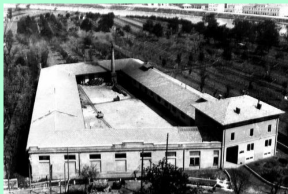
8. View of the metallurgical factory, 1931
