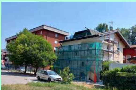
6. Small construction site of building in Doss Trento street
