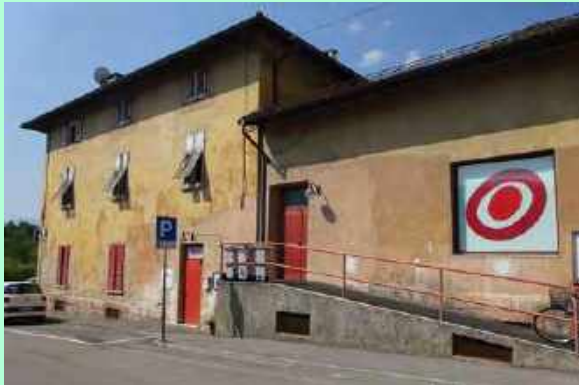
5. Portland Theatre in Papiria Street
