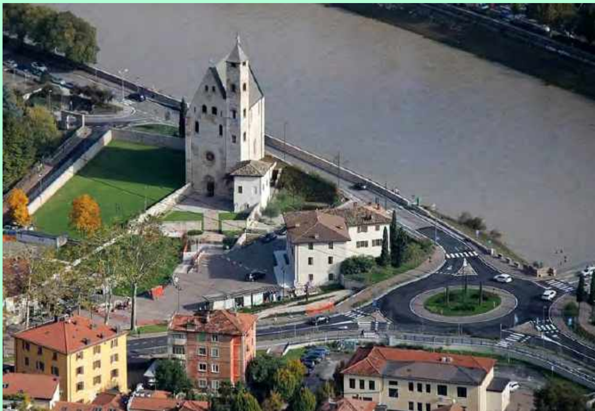
1. View of new roundabout
