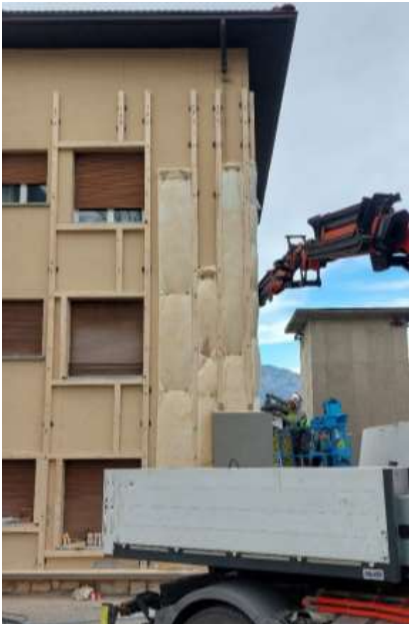
Figure 56. Installation of the Renew Wall panels. Source: UNITN.
