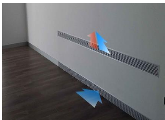
Figure 126. Wall-mounted fan coil (source: JAGA).
