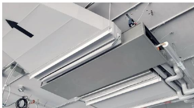
Figure 125. Installation of ceiling fan coils (source: JAGA).
