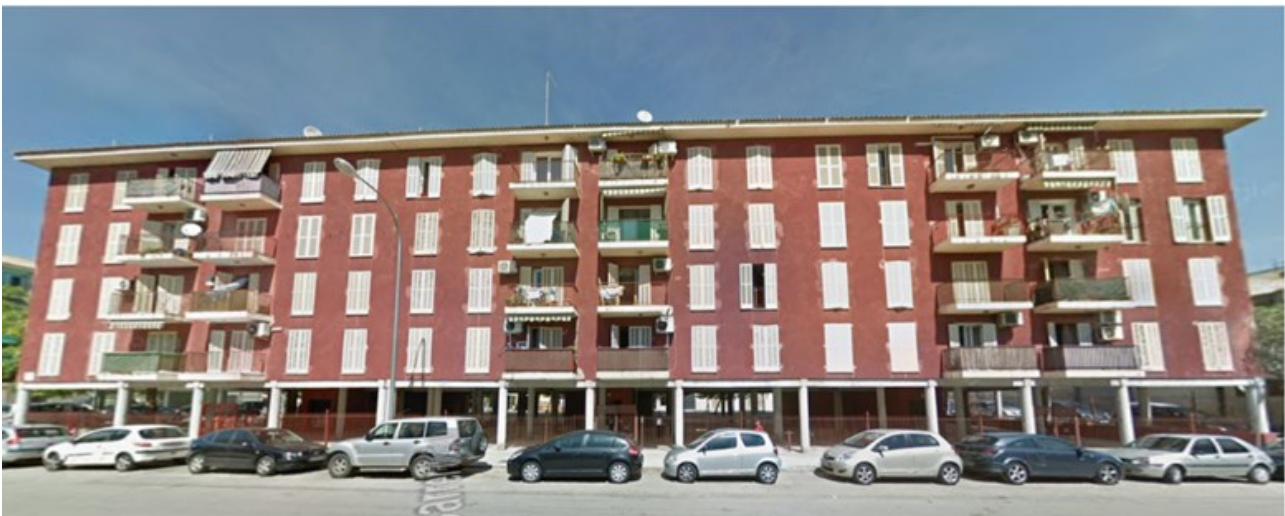
Figure 11. Selected building archetype for the renovation: large multifamily building.
