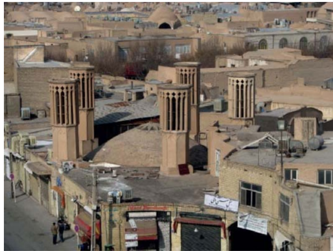
Figure 14: Yazd (Iran) – traditional wind towers [25]
