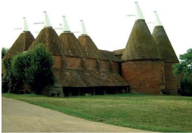
Figure 18: Wind cowls able to move with the wind changing direction in a beer brewing of Kent (England) [25]
