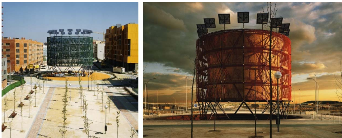
Figure 1: “Ecobulevar de Vallecas” in Madrid (Spain). Built from recycled plants and materials, the building is able to lower the temperature by up to 10 °C by mimicking a greenhouse system [7], [12]
