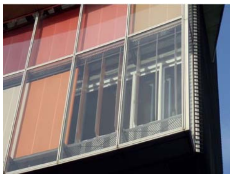
Figure 27: GSW building in Berlin (Germany) – cross ventilation is facilitated by the double glass façade providing a stack [25]
