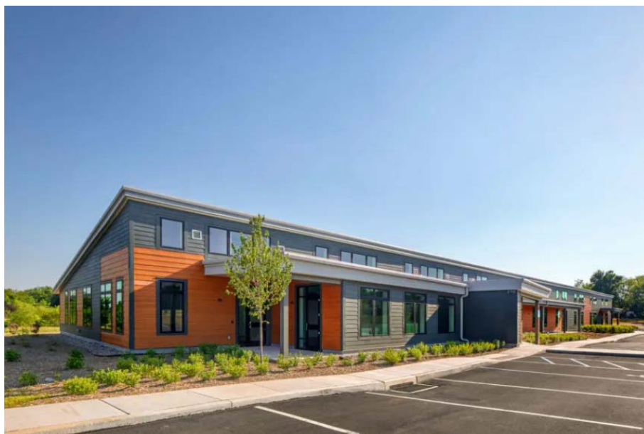
Figure 4: “Sustainable Energy Fund Office Building” in Schnecksville (Pennsylvania, USA). The building orientation and windows’ design allows to take advantage from shade, sun and daylight, minimizing the loss of energy. It also uses a roof photovoltaic array. It is planned to generate 130 % of the required energy [15]
