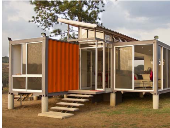
Figure 25: Openings on opposite sides and at different heights of a space, allowing cross and stack ventilation [32]
