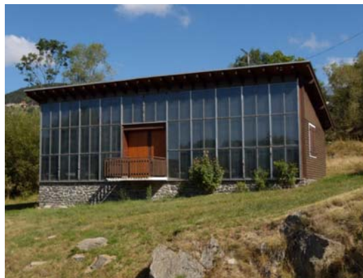
Figure 29: Trombe wall in Vivienda Trombe (Odeillo, France) [34]
