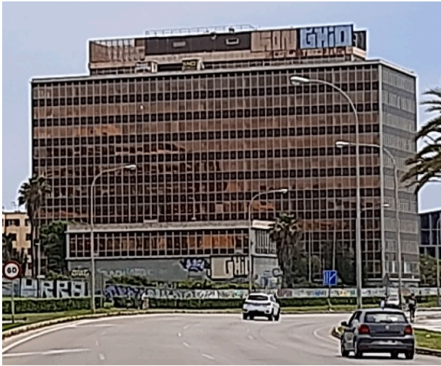
Fig. 1. Current state of the GESA building, picture by authors.
