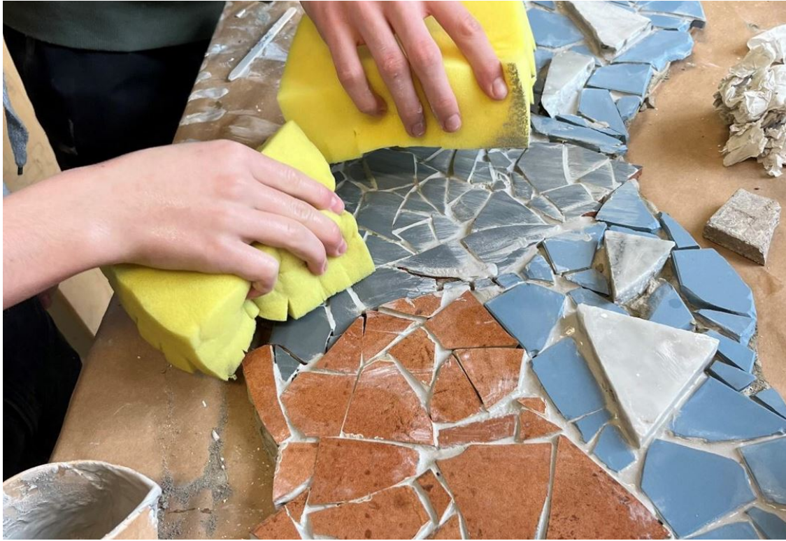
It's important to remove the grouting from the tile surfaces! Photo: SINTEF
