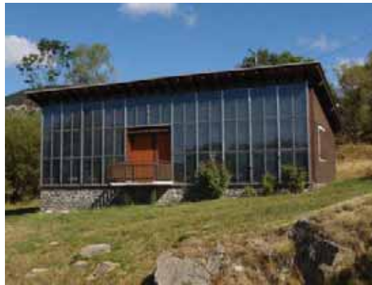
Figure 29: Trombe wall in Vivienda Trombe (Odeillo, France) [34]
