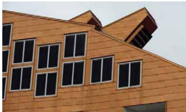
Figure 22: Harm A. Weber Academic Center at Judson University in Elgin (Illinois, USA) – ventilation exhaust device on the roof [25]
