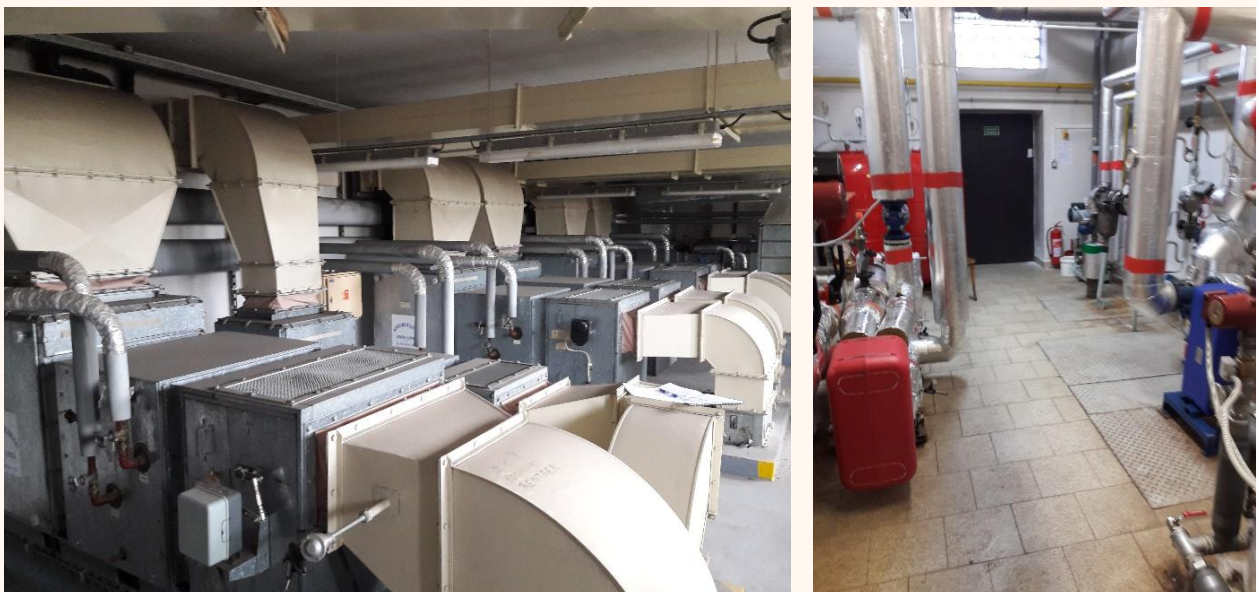
Figure 22. Current status of the HVAC system in the building. The heat exchange station is modern and operated by third party.
