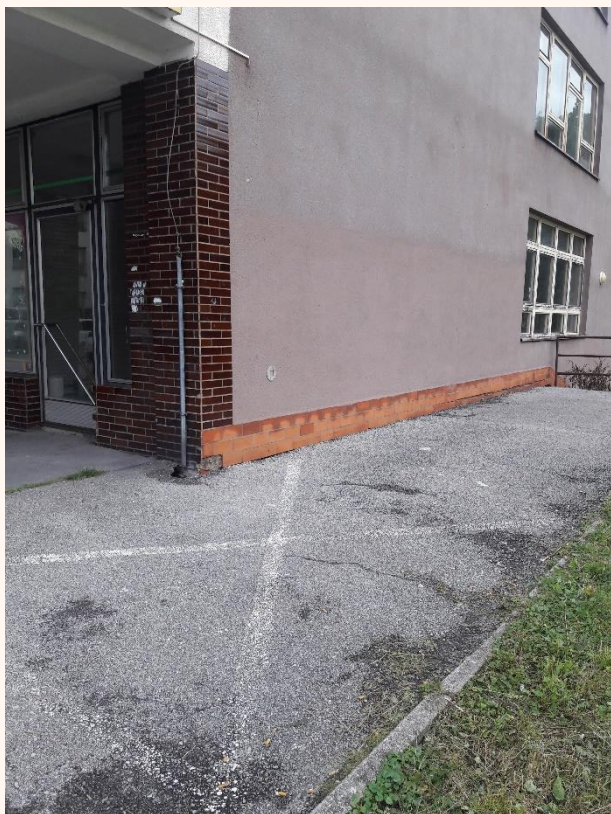
Figure 16. Current status of the ground floor structures with significant moisture transport in the left and typical obsolete window in detail in the right.
