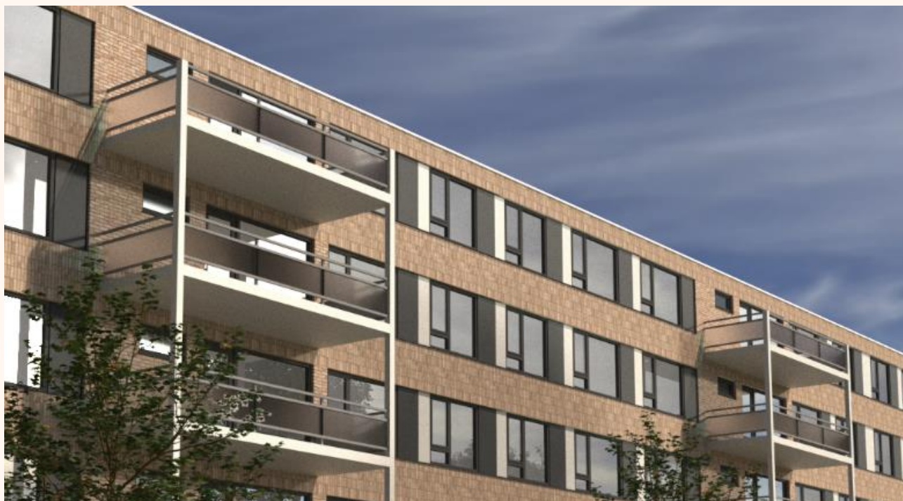
Figure 24. 3D presentation of the front façade of a renovated Bredero building
