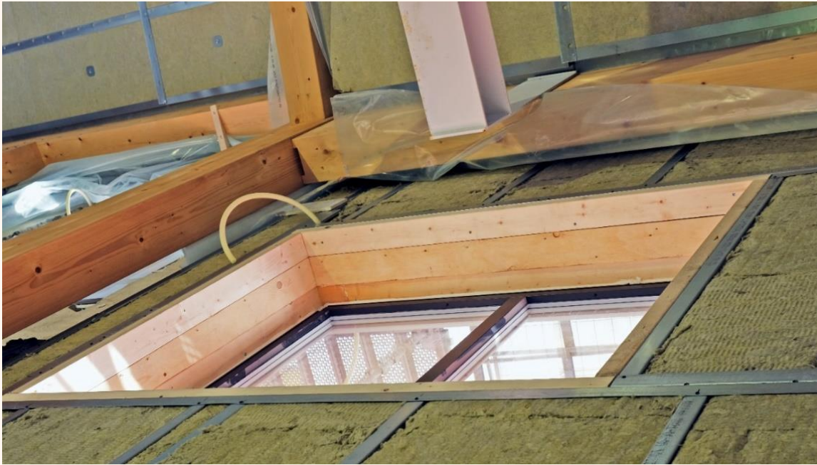
Figure 33. Image of the internal insulation layer in the H-building. The new wood structural system is shown. The gypsum boards, not installed yet, are to be placed between the vertical and the horizontal wood frame. Photo by Nicola Lolli (SINTEF).
