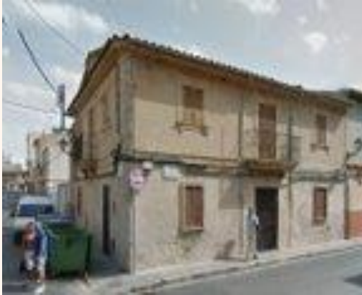
Figure 16. The one-stop-shop renovation project at the centre of activities (picture of building before renovation).
